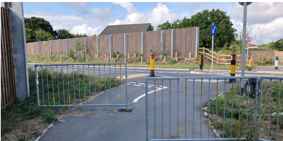
Image 3.2: Brookers Lane / Woodcote Lane footway cycleway
